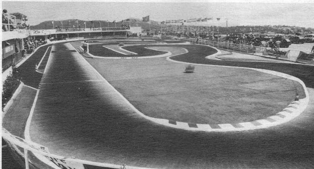
Below: a prime example of the circuit constructor's art. This one is situated at Carnoux, Southern France and was the venue for the 1983 World Championship event.
